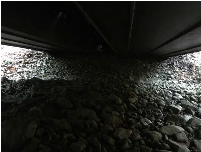
Left Bank Abutment when facing downstream
